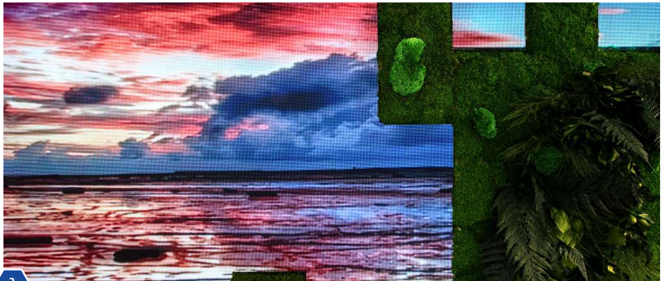
2 Close up of LED wall integrated with live moss wall
